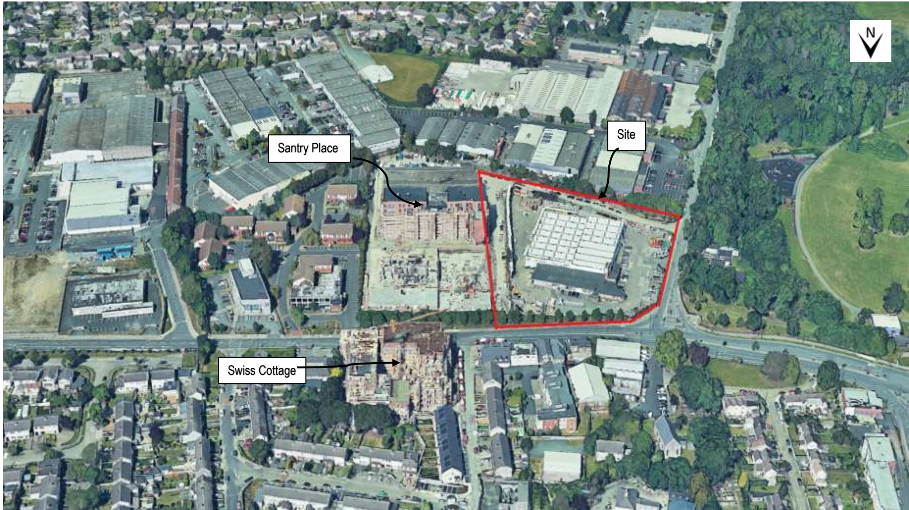
Figure 3 – Aerial View of Subject Site, looking from west to east.
